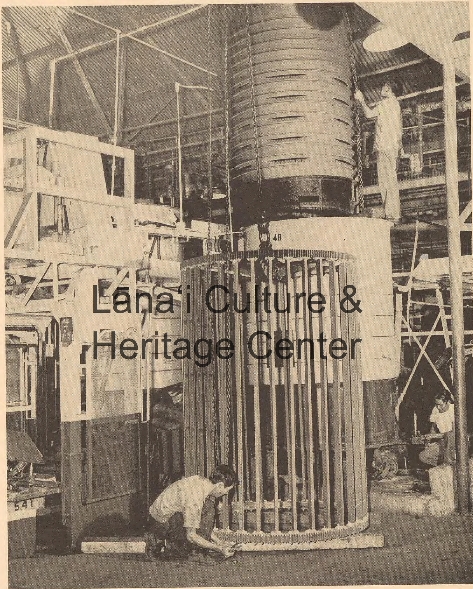
COMPLETE OVERHAUL of huge can coolers is made after peak canning season slacks off. One by one, each of the line of more than forty of these machines is taken apart, thoroughly cleaned of any rust and dirt, painted inside and out, and put back together again, ready for another year of use. Cleaning and checking of each cooler takes three men about fifteen days. This one will hold 556 cans at one time, and the largest has a capacity of 765. Tadao Tukuda, left, Wah But Shun, standing on the tank, and Segundo Rodolfo, right, check carefully to avoid costly breakdowns during the next season.
