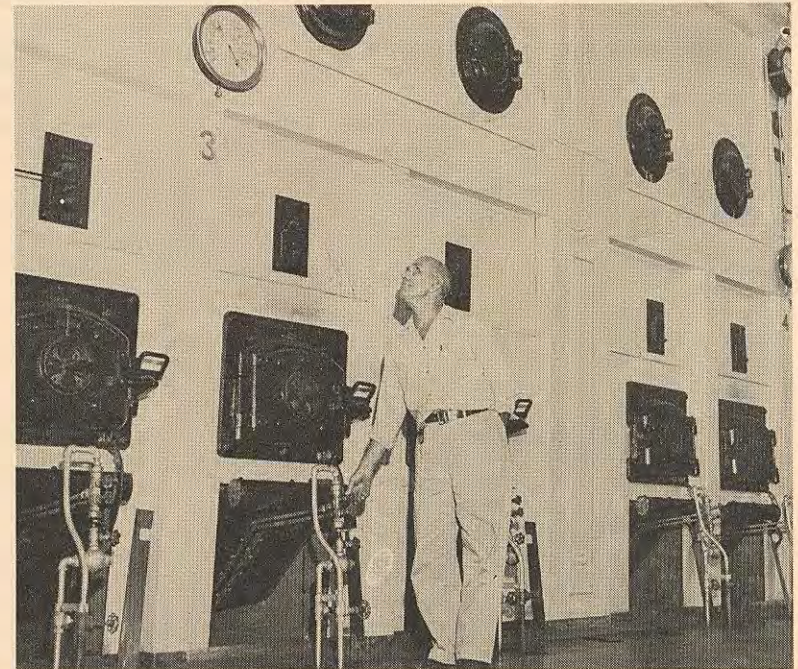
HUGE PUMPS AND BOILERS keep steam ready for its many uses in the cannery. Kazumi Tagawa, above left, checks pumps that bring fuel oil from supply tanks into fire room and to burners. At right above, John Souza watches to see that pressure is kept at 110 lbs. In peak season, 14 to 15,000 gals. of crude oil per day are used, and boilers put out over 2,000,000 lbs. of steam.
